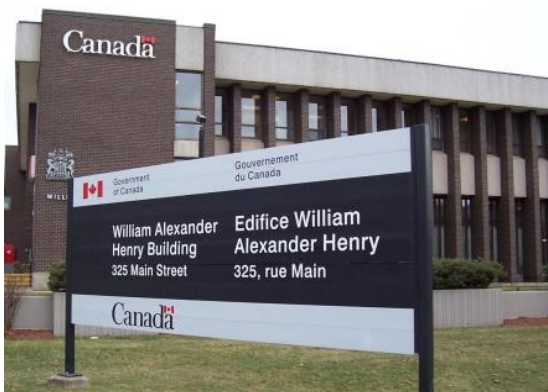
Service Canada Building in Antigonish
